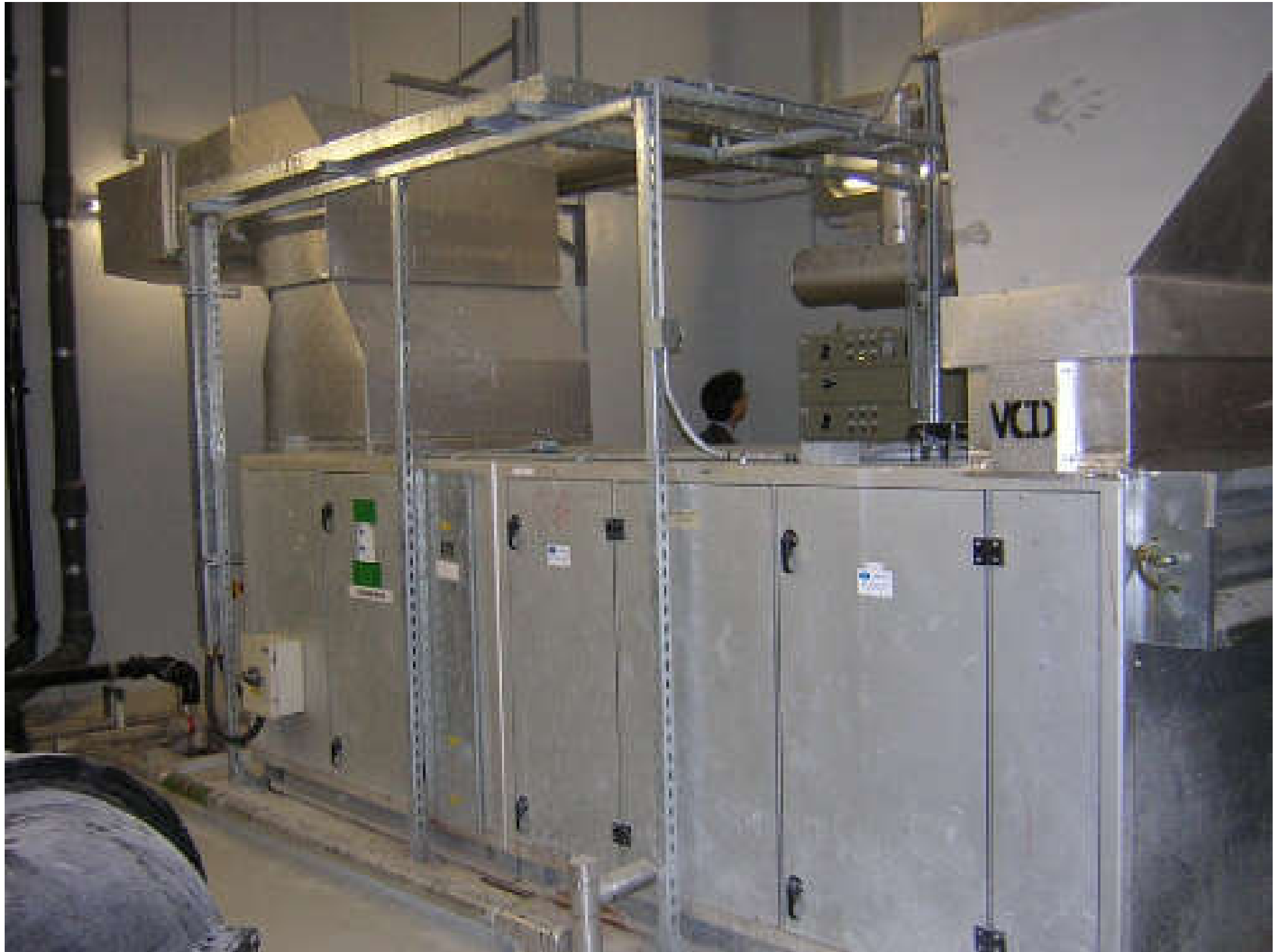
Example of an air-handling unit (modular type)
