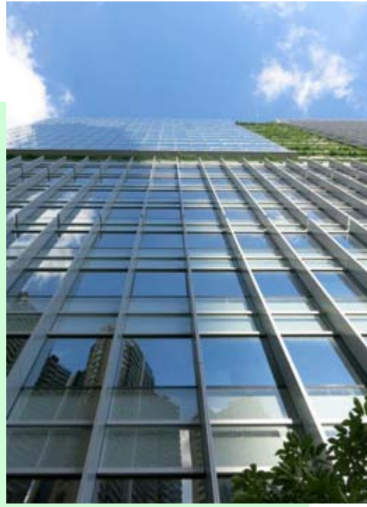
Close up of the vertical sunshades (left) and application of sunshades in different areas of the façade (right) to reduce heat gain and glare.
