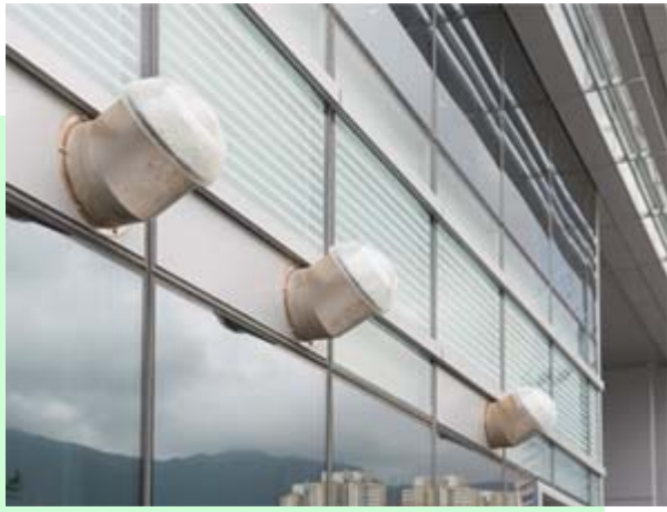
Photo showing the anidolic light pipes in the façade for Building Management Office (left). Diagram showing the anidolic light pipes (right), configured to transmit sunlight horizontally.
