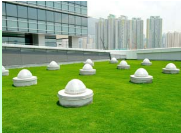
Sun pipes transmit sunlight from the roof of the community hall (left) through high reflective internal surfaces to the multi-purpose hall (right)
