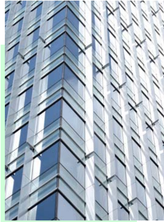
Close up of the vertical sunshades (left) and application of sunshades in different areas of the façade (right) to reduce heat gain and glare.
