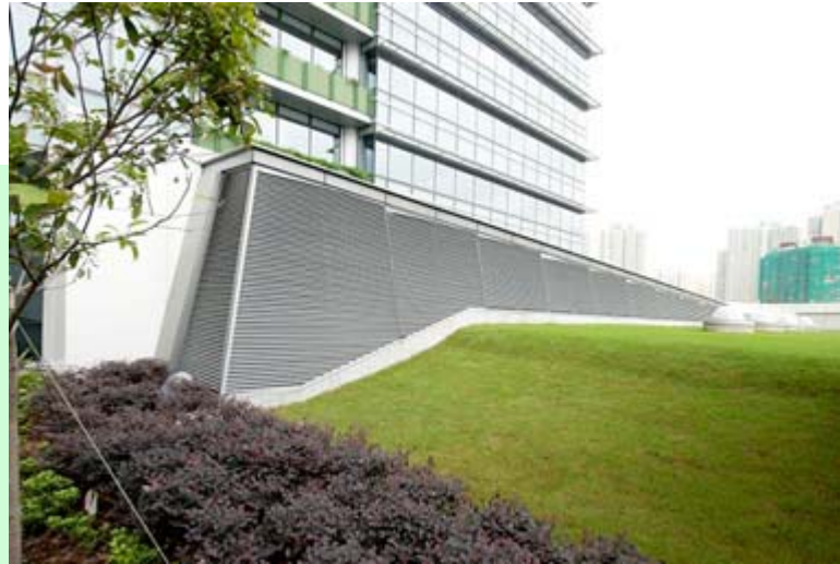
Outlet of the solar chimney in the community hall roof
