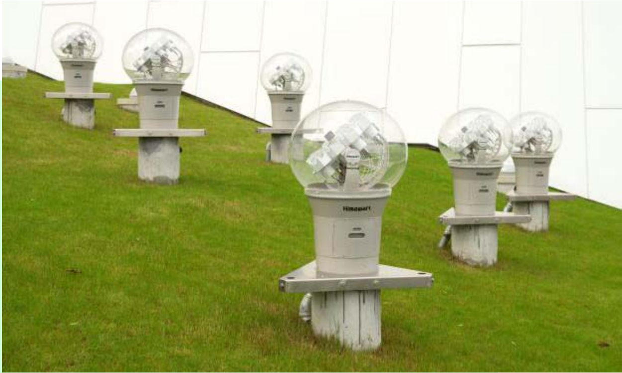
Solar Tracking Optic Fibre Light Pipes maximise sunlight collection by use of automatic solar tracking devices
