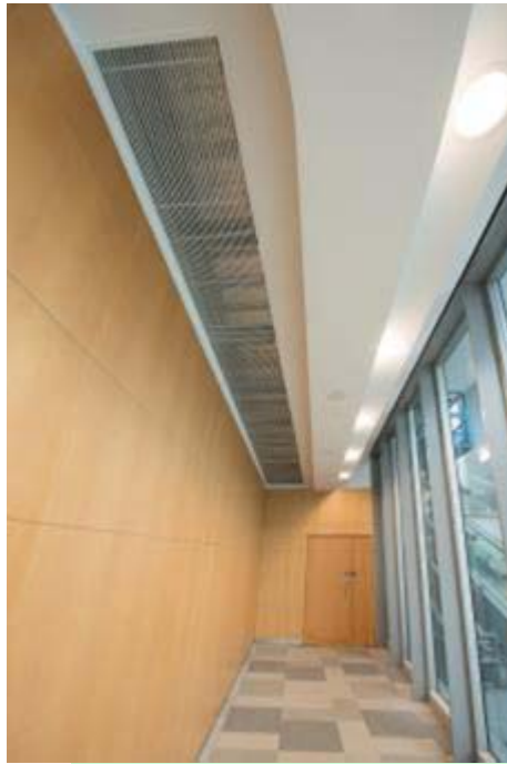
Solar chimney in the community hall foyer
