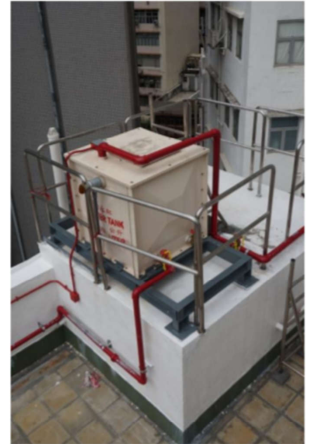
Supply Tank of 500-litre installed on Roof-floor
