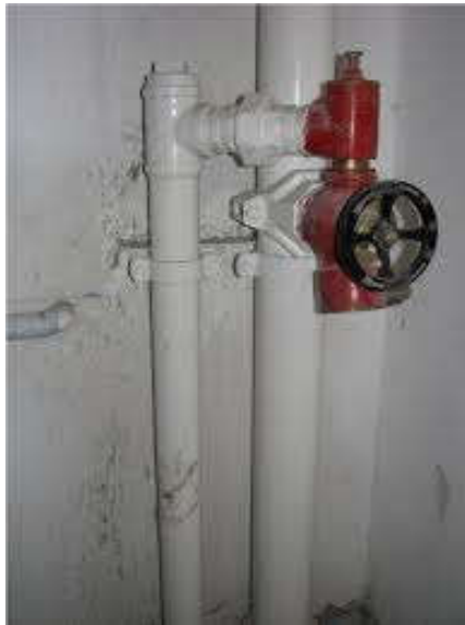
Fire Hydrant – Single Outlet with Parity Valve
