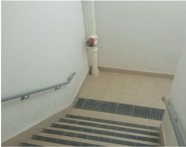
Fire Hydrant in Staircase
