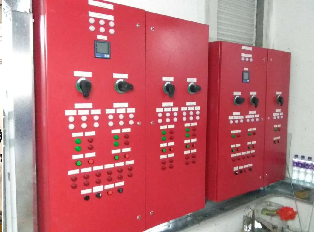
Fire Services Pump Control Panel
