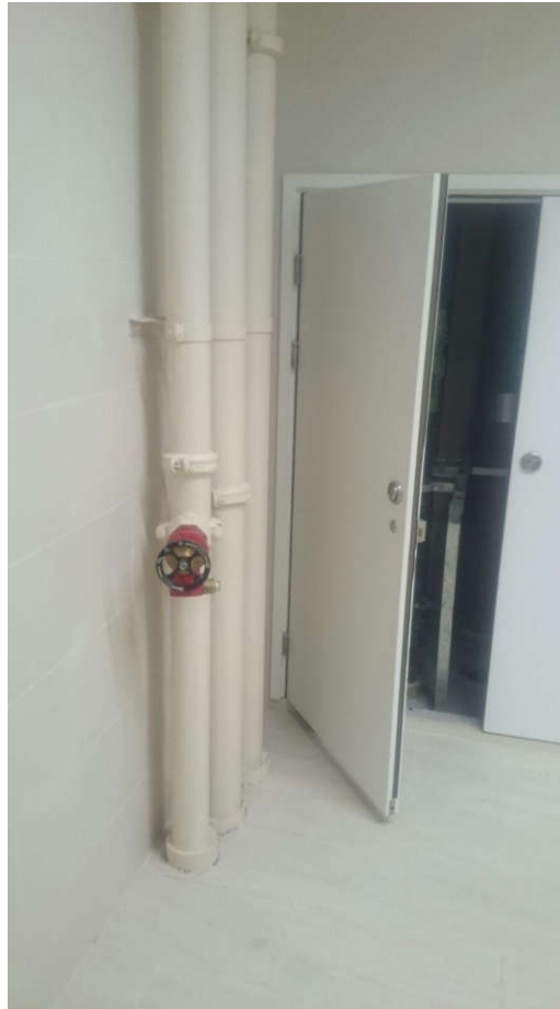
Fire Hydrant in Protected Corridor
