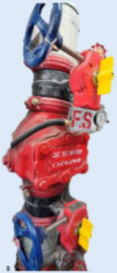
Sprinkler Control Valve
