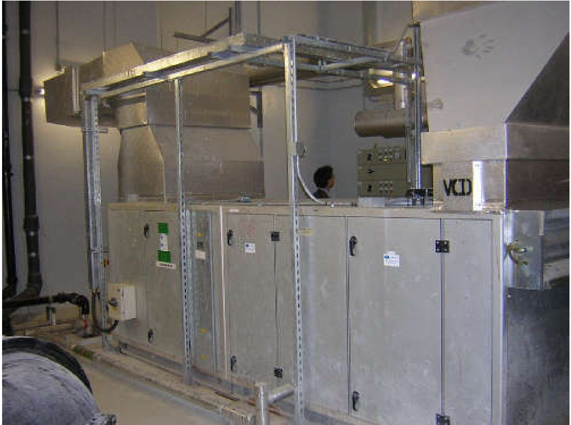
Example of an air-handling unit (modular type)
