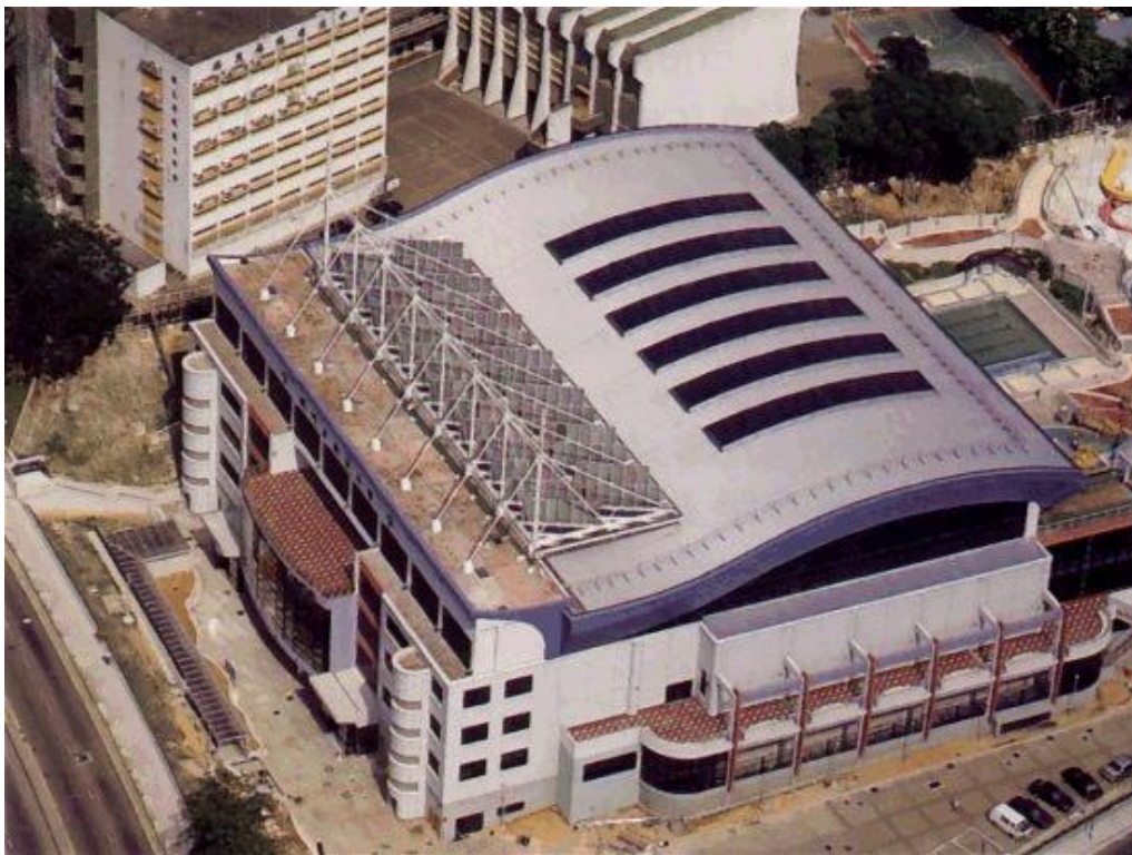
Solar heating for a swimming pool complex in Kwai Chung (313 sq.m solar collectors)
