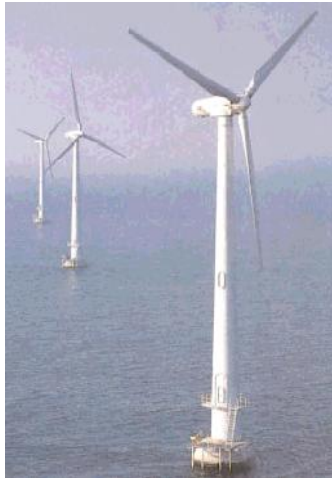
Off-shore wind turbines
