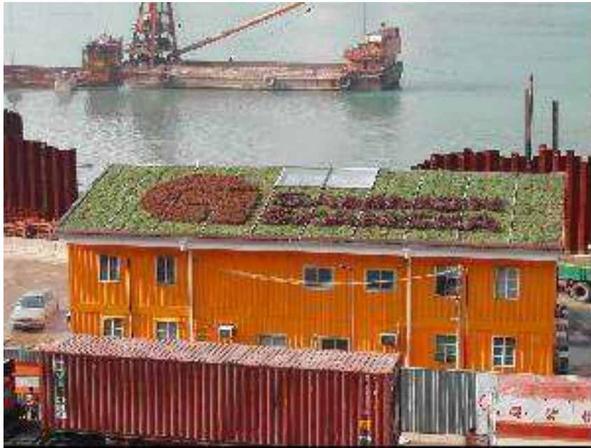
Green site office
