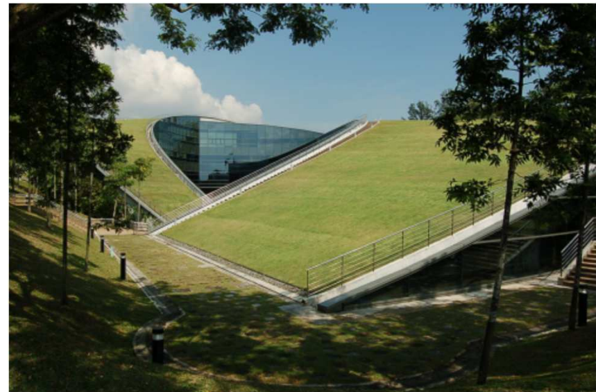
Lawn green roof (Nanyang Techn. Univ.)
