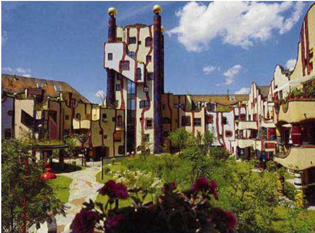
Green roofs in Germany (2000) (Hundertwasser Building, Darmstadt)
