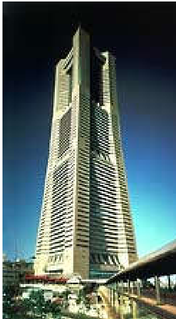
Landmark Tower, Yokohama, Japan (max. lift speed 750 m/min or 12.5 m/s)
