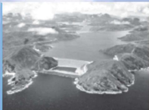
1978 Completion of High Island Scheme 281 mcm capacity
