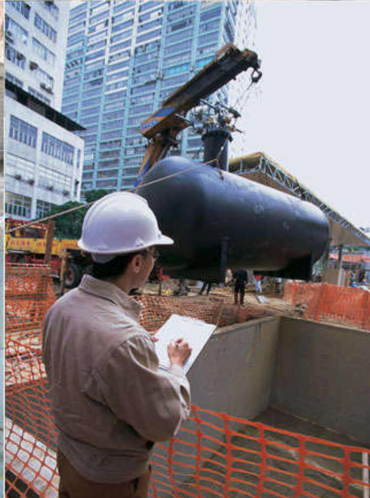
Central LPG storage installation
