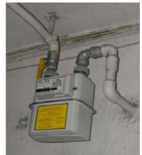
Figure 3: An installation pipe and gas fittings
