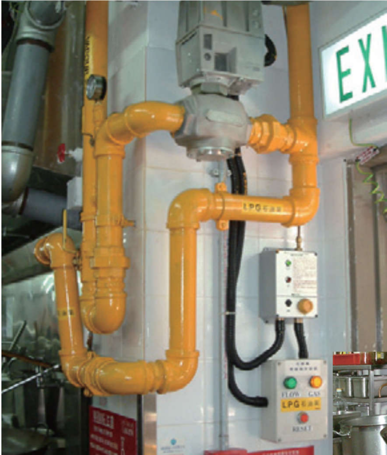
Control valve & meter
