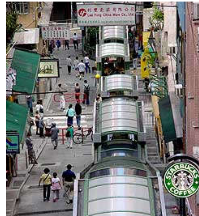
Central-Mid-Levels Escalator, total 790 m
