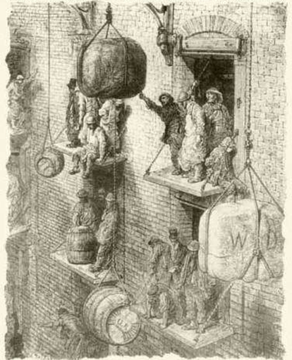
The London Dockyards comprised warehouses virtually forming a five or six-story wall along the Thames River. A centrally located steam engine usually provided power to upper-floor "transporter" hoists that raised and lowered goods on one side of a building and similarly served land transport on the reverse side. Many such hoists had the dual purpose of running loads in and out of the warehouse from window loading ledges.
