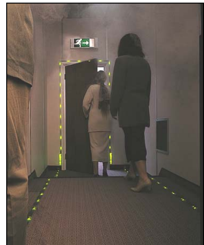
Fig 23 Low location lighting
