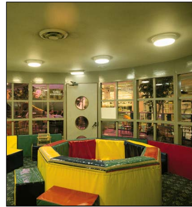
Fig 3 School with emergency lighting
