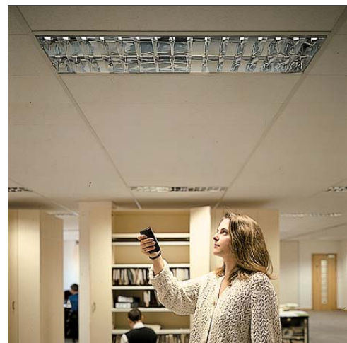
Fig 9 Use of remote control to set luminaire
