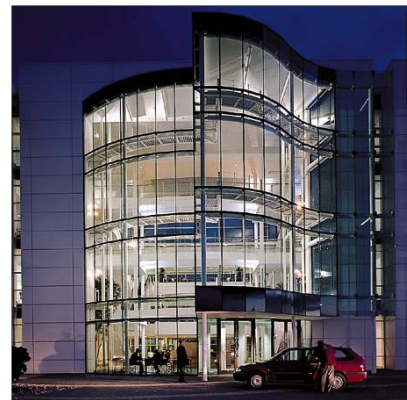
Fig 10 Lighting usage is very visible
