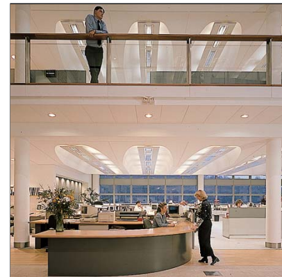
Fig 7 Lighting in barrel vaults
