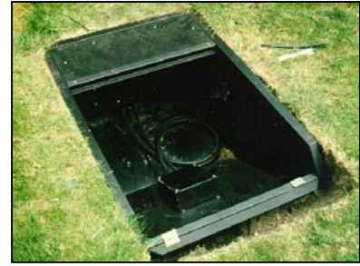
Fig 5 Recessed Ground Box during installation.
