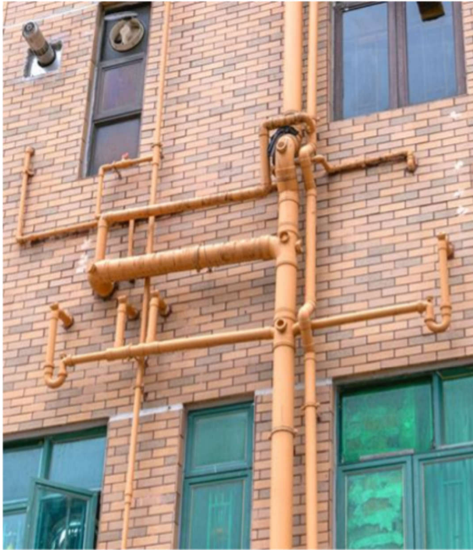
External wall of the building
