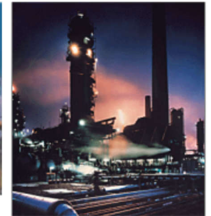
Petrochemical plant lighting
