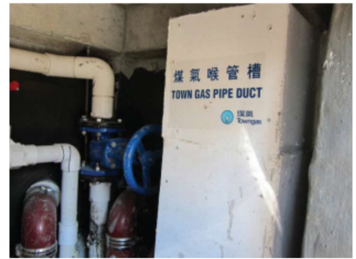
A town gas pipe duct
