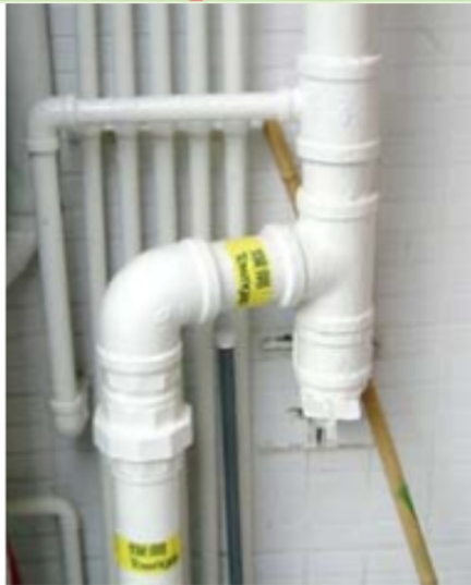
Figure 1: Vertical sections of a service riser
