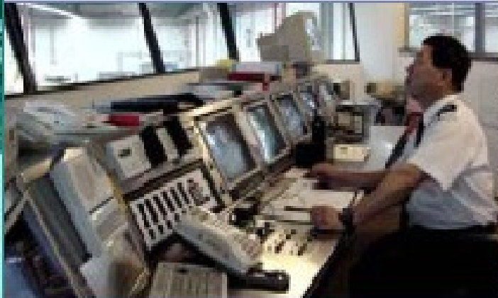
Security control centre
