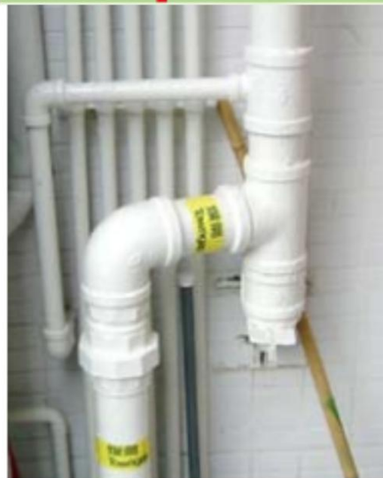
Figure 1: Vertical sections of a service riser
