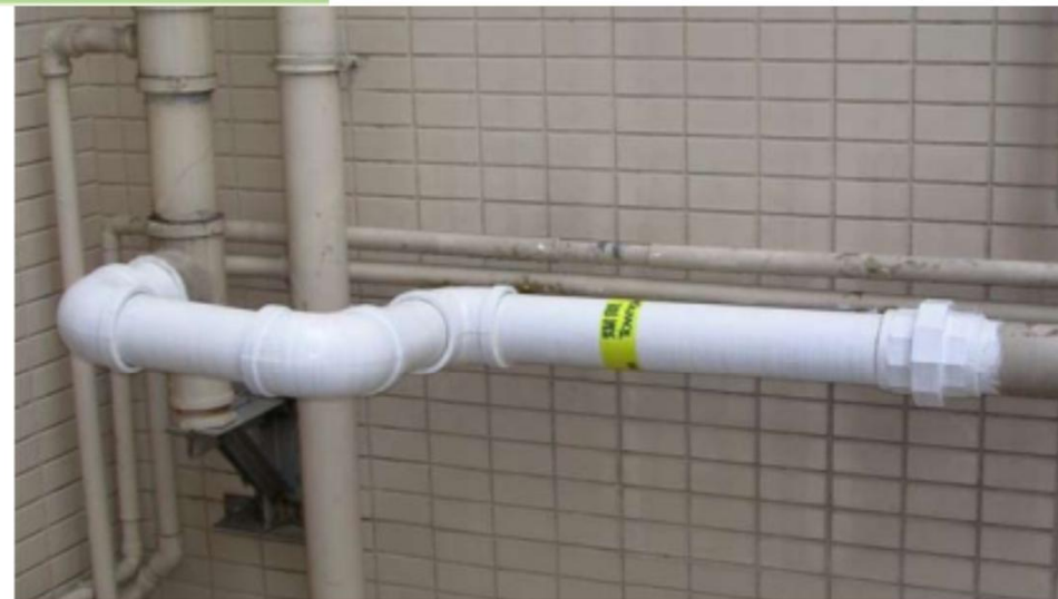
Figure 2: Horizontal sections of a service riser
