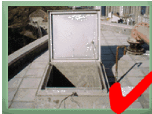
Double sealed tank cover with lock
