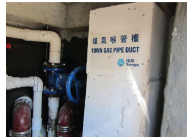
A town gas pipe duct
