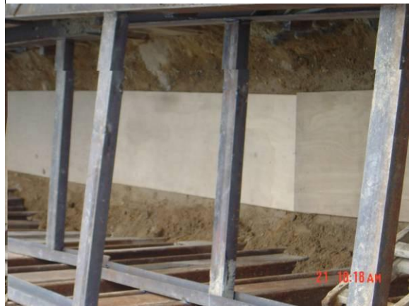
Fig. 5.8 Finished first layer backfill
