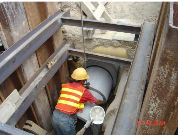
Fig. 5.5 Set pipe in position by crane
