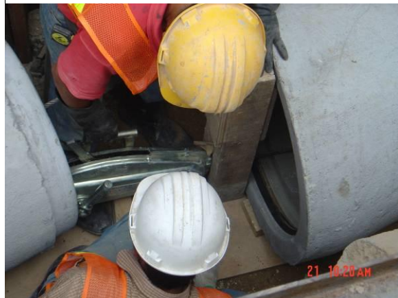
Fig. 5.6 Pipe re-position by manual tool
