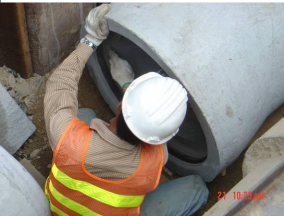
Fig. 5.7 Setting of rubber ring
