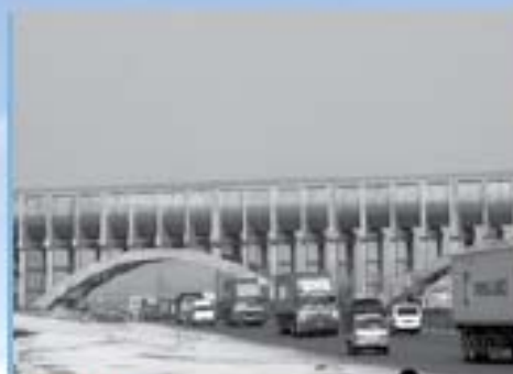
2003 Commissioning of 83km dedicated aqueduct for delivery of Dongjiang water
