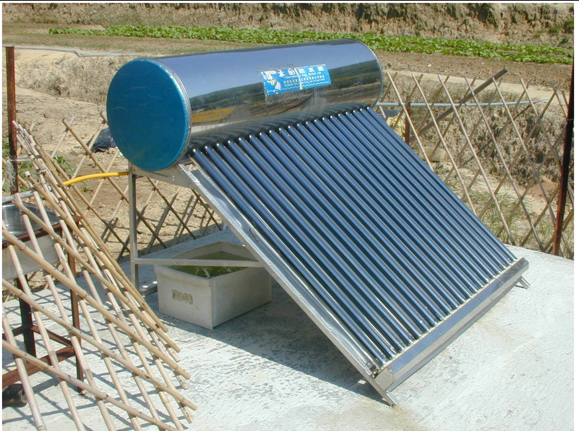
Evacuated-tube solar hot water system
