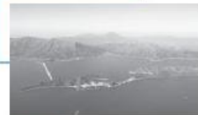
1968 Completion of Plover Cove Scheme and Extension in 1973 230 mcm capacity
