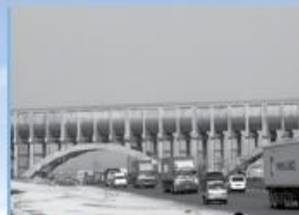
2003 Commissioning of 83km dedicated aqueduct for delivery of Dongjiang water
