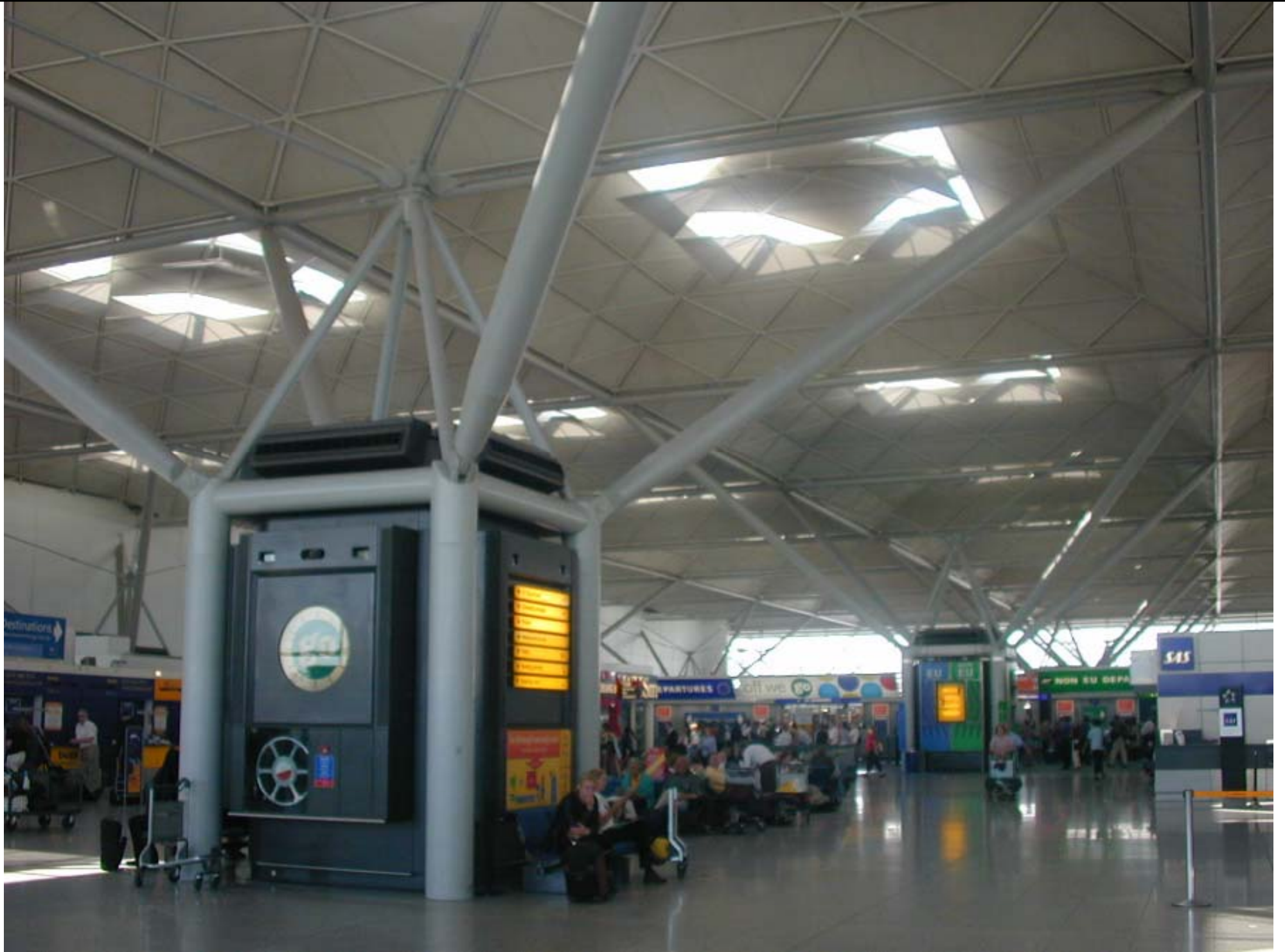
Stansted Airport, UK
