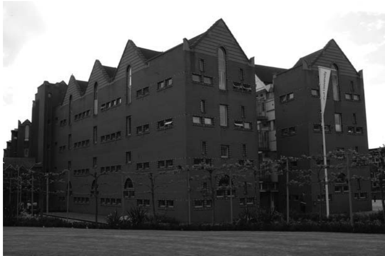
FIG 15.13 Queen's Building at De Montfort University, Leicester.
