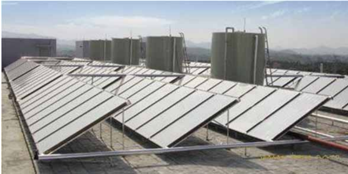
Flat-plate solar collector
