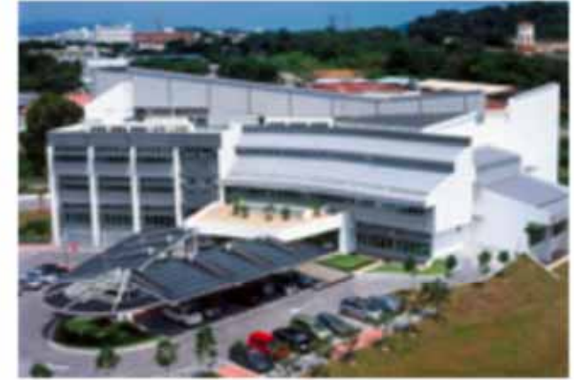
Pusat Tenaga Malaysia's ZEO Building, Malaysia [2007]
