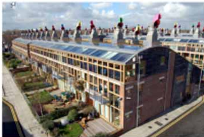
Beddington Zero Energy Development (BedZED), London [2002]
