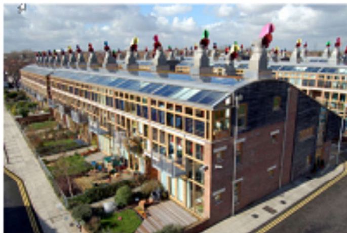
Beddington Zero Energy Development (BedZED), London [2002]
