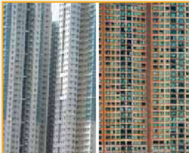
Wall-like barriers causing negative visual impact and reducing air flow
