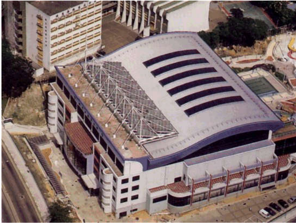
Solar heating for a swimming pool complex in Kwai Chung (313 sq.m solar collectors)
