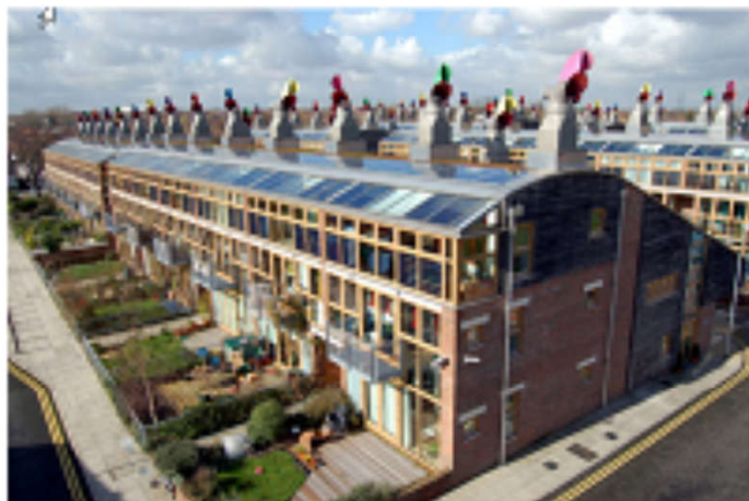
Beddington Zero Energy Development (BedZED), London [2002]
