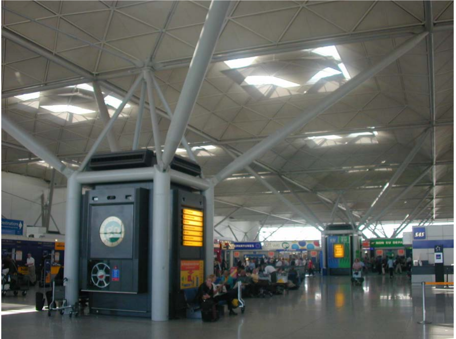
Stansted Airport, UK
