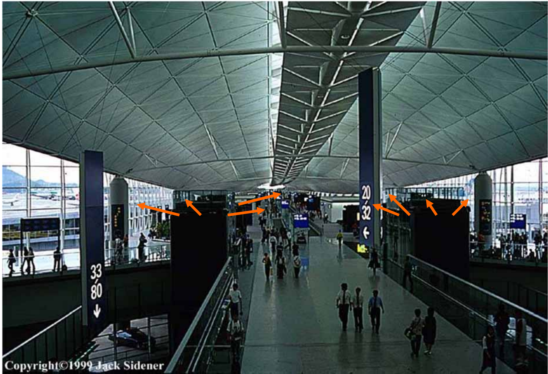
Hong Kong International Airport
