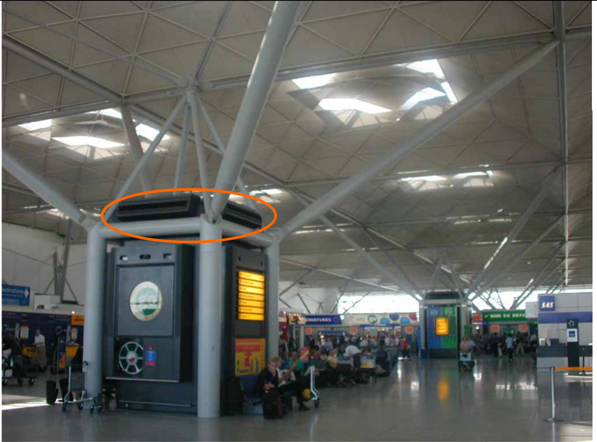
Stansted Airport, UK
