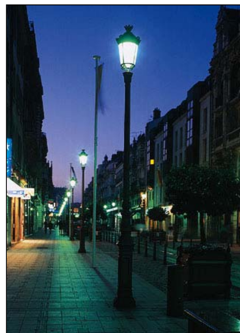
Fig 66 MBF lamps used in amenity lighting.
