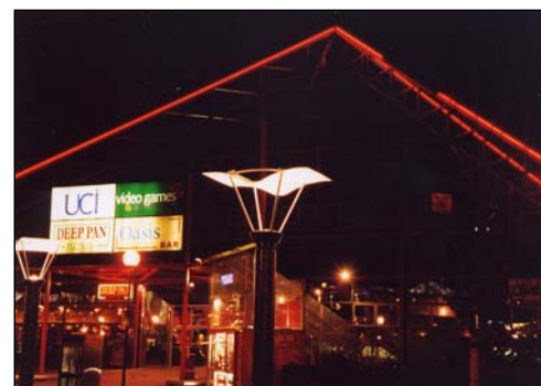
Fig 38 Red cold cathode installation.
