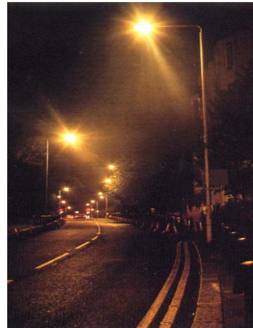
Fig 59 SOX lamp road lighting.
