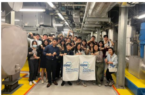
Technical Visit to Chiller Plant at Swire Taikoo Place (SA x YEA) on 29 Oct 2024
