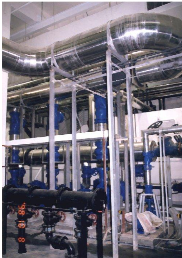
Solar hot water pumps and water filtration plant room [at basement] of the swimming pool
