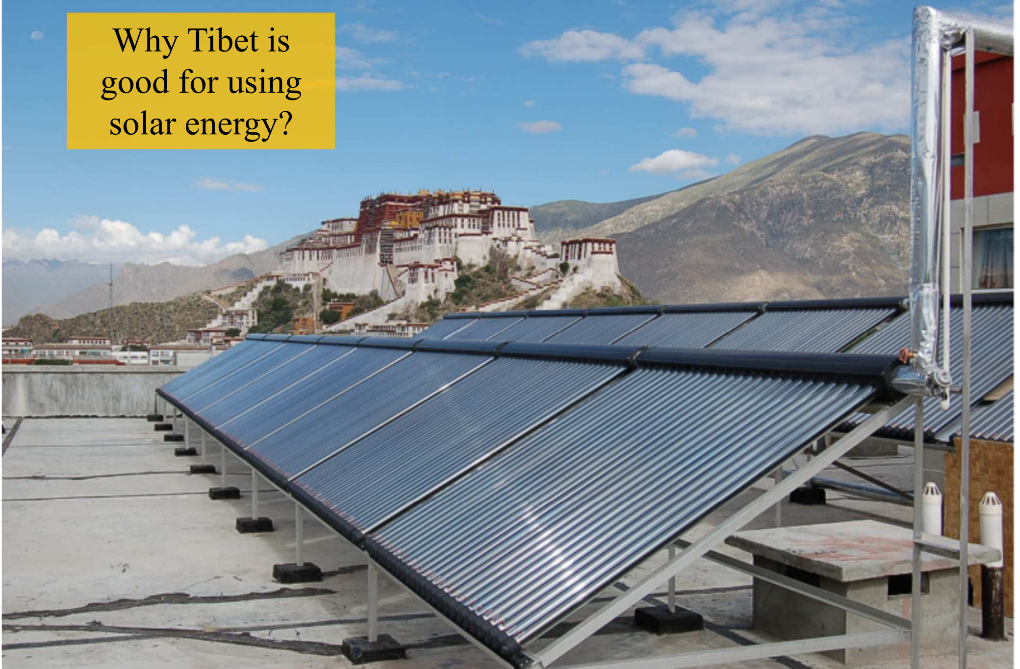
Evacuated-tube solar hot water system in a hotel in Lhasa, Tibet (photo taken by Dr Sam C M Hui)
