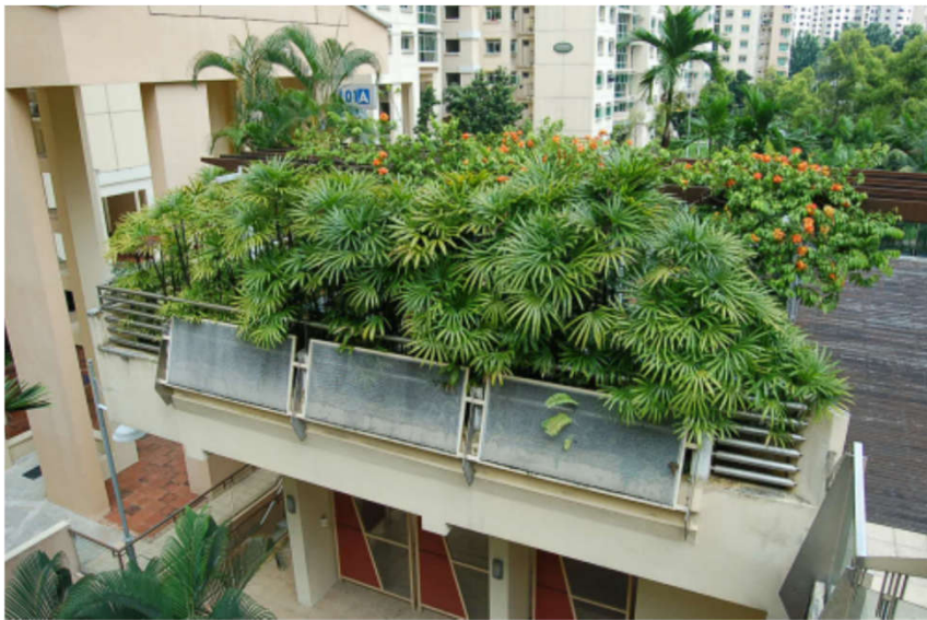
Carpark roof of public housing (intensive green roof)
