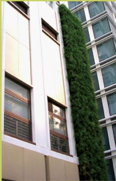
Figure 6 The signature vertical green wall at 2/F
