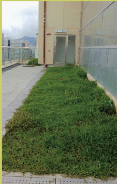
Figure 7 Part of the green area on the roof
