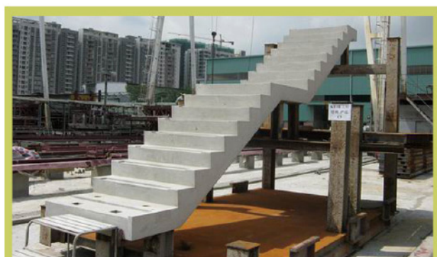
Figure 21 A precast staircase
