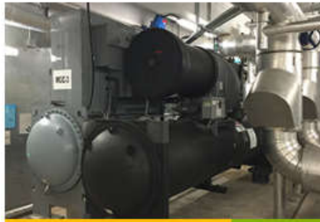
Water-cooled air-conditioning systems
