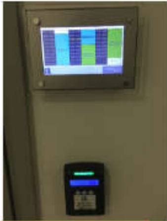
Automatic on-off for lighting and fan coil units in classrooms
