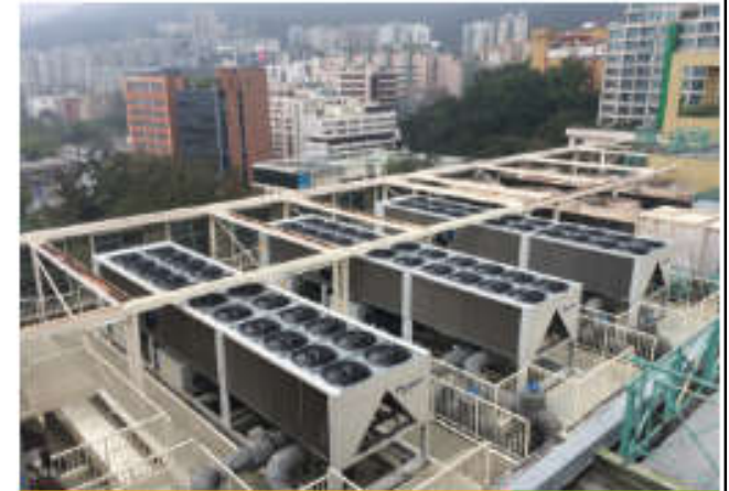
Replacement of existing chillers with better energy performance options
