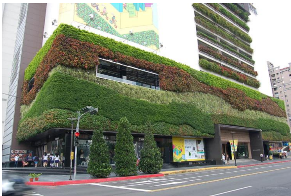
(a) Outdoor green wall (Taichung, Taiwan)
