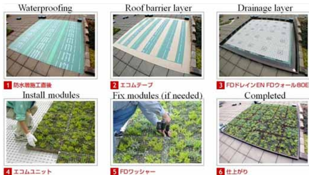
Figure 2.5 Installation sequence of a modular green roof system from Japan
