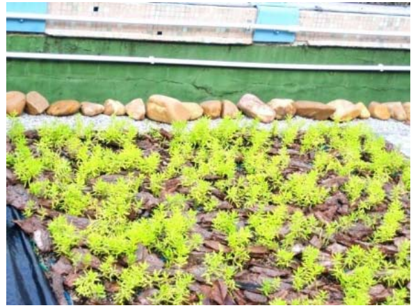
b) Sedum plant used on the green roof
