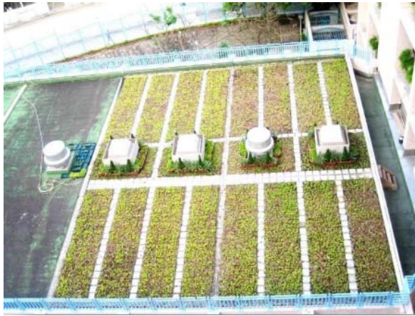
a) Overview of the green roof
