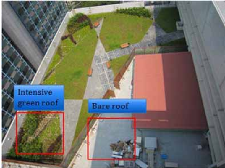
Figure 6. Measurement locations at a rooftop garden of HKU Main Library
