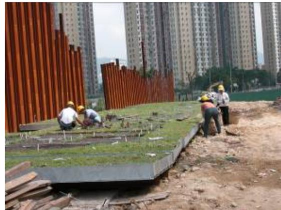
Figure 3. Modular design of the green roof system.
