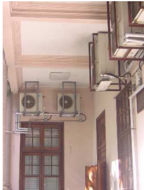
(b) Mounting of outdoor units for split-type units
