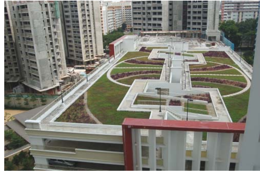
Carpark roof of housing estate (built-in green roof)
